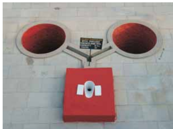
Sulabh twin-pit pour-flush compost toilet – a simple solution to achieve the Millennium Development Goal on Sanitation
