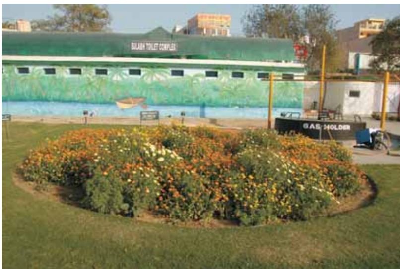
Biogas plant - Public toilets linked with biogas digester (with gas holder)
